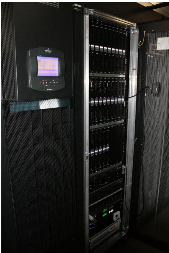
**Fig. 5** A view on some of **otto**'s components: Cooling rack (left), some computation nodes (upper right) and storage (lower right)
