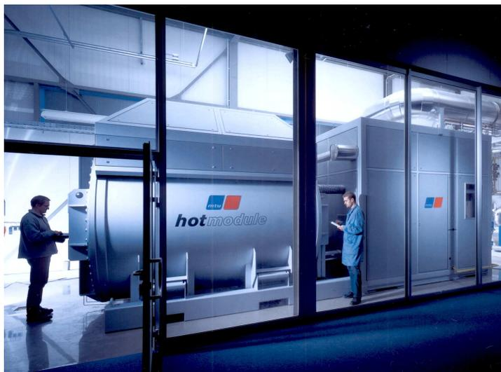
**Fig. 7:** The 200 kW MCFC stack HotModule at the Magdeburg university hospital operated by IPF Magdeburg and investigated within a joint research project funded by the BMBF.
